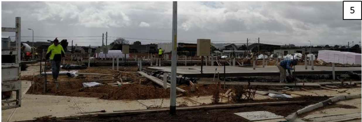
4. Stage 2 foundation works underway. 5. Stage 1 foundation works underway.
