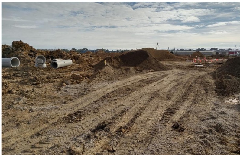
Entrance to Casey Green starting to take shape.
