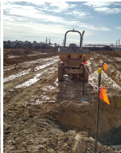
Roads being formed.
